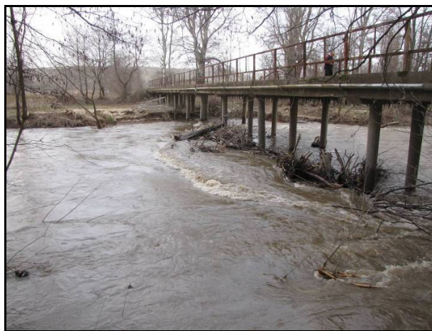
Figure 5. Huge quantity of deposits and vegetation debris in Pčinja River form dam-like barrier on the bridge, rising the river level upstream and leading to flood (19.02.2010). The bridge itself is in danger.
